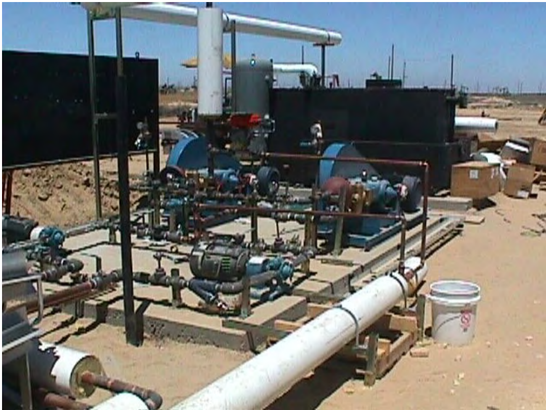
Figure 2.4-4. CO 2 injection pumps with heater in the background.
