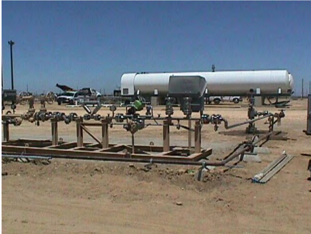
Figure 2.4-2. CO 2 Pilot Injection Header.
